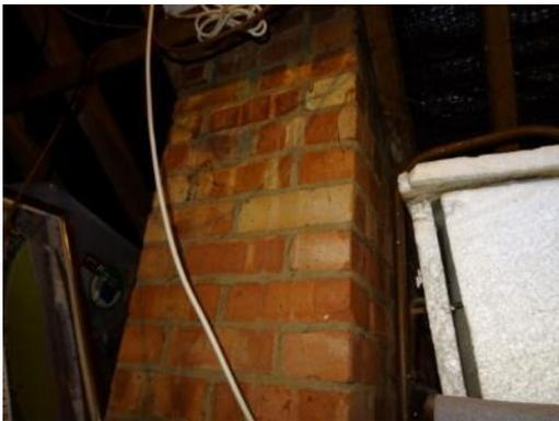
The cold water tanks are located within the roof void which are dated with the lids noted to be missing. Until such time that the cold water tanks are replaced, we would advise that the lids are reinstated in order to prevent vermin entering the tanks.
