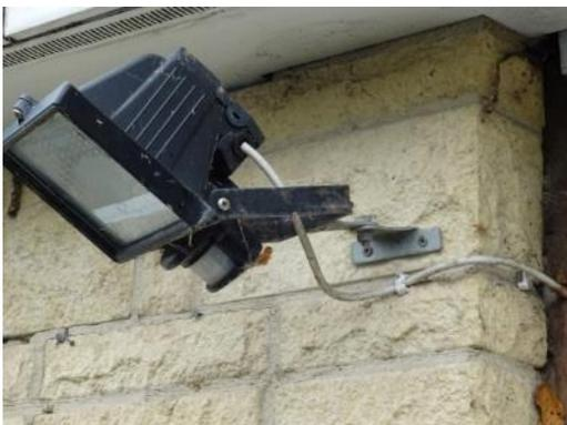
Minor localised repointing is required at high level adjacent the main entrance door. This is of no significant concern and simply a result of reverberation of heavy use of the door and
