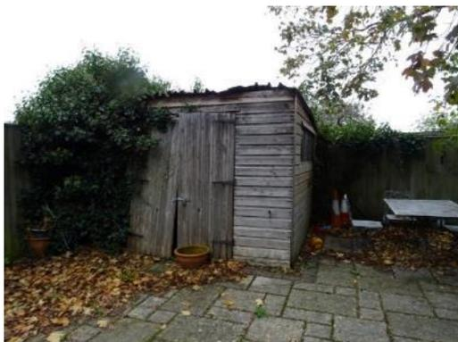
The boundaries around the garden are denoted by timber featheredge board with no significant damage noted. The fencing running along the left hand side of the garden was noted to be leaning over suggesting that the supports require replacing.
