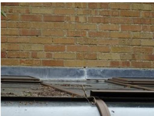
The conservatory has been seated on dwarf brick walls. Various bricks were noted to have debonded therefore will require localised re-building at the time the conservatory is replaced.
