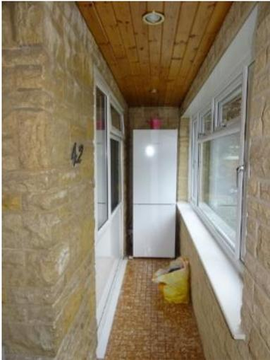
The ceiling has been formed in timber panelling, which is relatively dated, therefore you may wish to consider removing this at which time the ceiling will require plasterboard and skimming.
