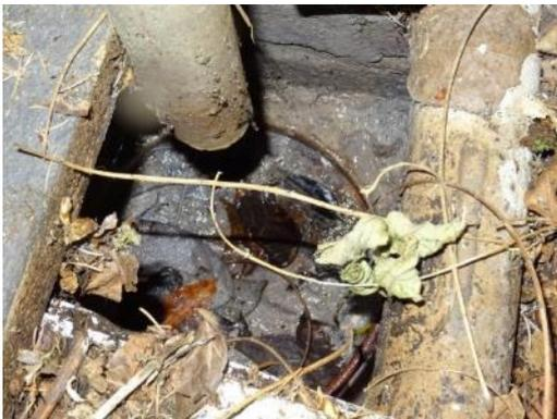
A redundant wastepipe is located to the right hand side of the elevation which we would advise is removed with the opening then filled in order to prevent risk of vermin ingress.
