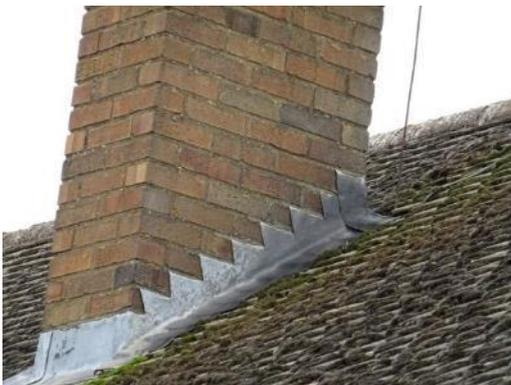
The roof covering is in a serviceable condition with no slippage or deterioration of the tiles noted.
