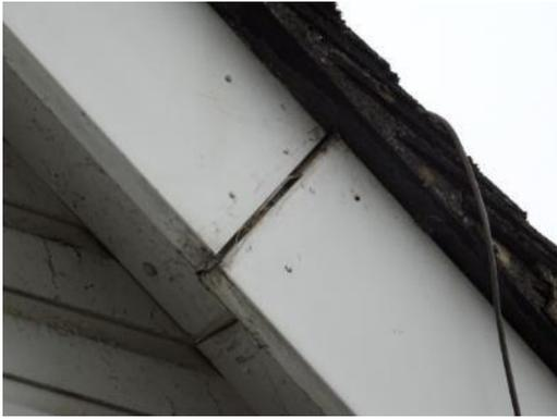
The soffits to the underside of the roofs are uPVC which are noted to be pulling away requiring re-securing into position until such time that the soffits are replaced.
