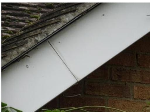
The dormer gables and cheeks have been finished with uPVC panelling, which is relatively begrimed requiring cleaning down however is considered serviceable having been firmly secured into position. Minor localised damage was noted to the uPVC capping above the right hand dormer window which is of no significant concern.
