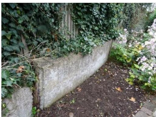
It should be noted that we consider the concrete walls to be retaining, therefore will require reconstruction at the time of demolition.
