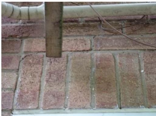
Staining was noted to the brickwork beneath the snug window where the gutters were noted to be overflowing. Once it can be confirmed that the gutters are free flowing, we would then advise that the brickwork is cleaned with a soft wire brush.
