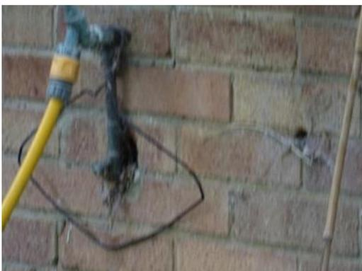
The wastepipe serving the kitchen discharged over an open gulley which was noted to be defective. We would advise that the open gulley is replaced with a proprietary unit in order to prevent risk of escape of water around the gulley.
