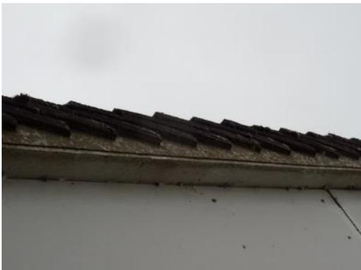
The soffits and fascias are uPVC which have been amateurishly installed but are considered fit for purpose and firmly secured into position.
