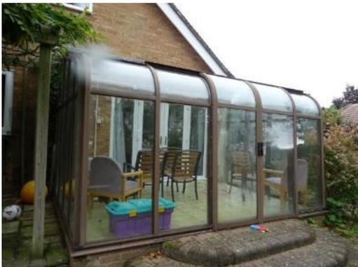
Where the conservatory abuts the main body of the property, lead flashings have been installed with the lead noted to be in a serviceable condition and firmly dressed into the brickwork.
