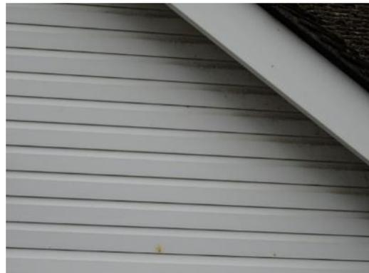
Various junction caps were noted to be missing which we would advise are replaced in the immediate term in order to prevent risk of water ingress in times of wind driven rain.
