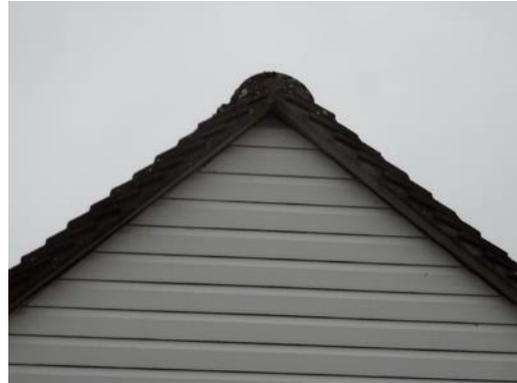
The tile under cloak appears to have been formed in fibrous board. It should be noted that fibrous board in properties of this age and type may contain asbestos. Therefore, should the fibrous board be disturbed, we would advise that it is tested with specialist precautions taken if necessary.
