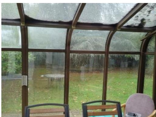
Localised damp staining was noted to the underside of the skylights where we consider the seals to have failed.
