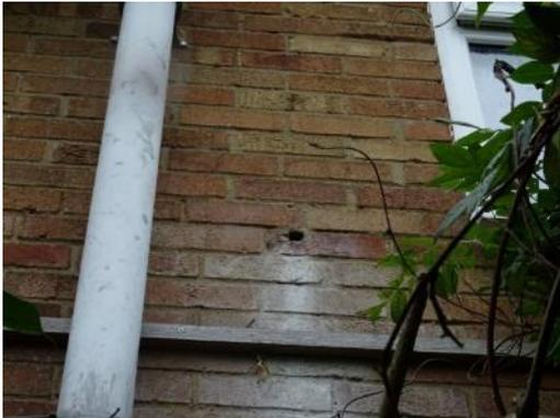
The mastic seal around the edge of the window frames is in a deteriorating condition requiring cutting out and renewing.
