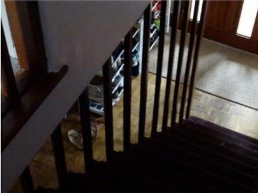
The staircase does not finish flush with the wall and we consider this an area where injury could occur. We would therefore advise that a stair stringer is installed in order for the gaps to be no greater than 100 mm.
