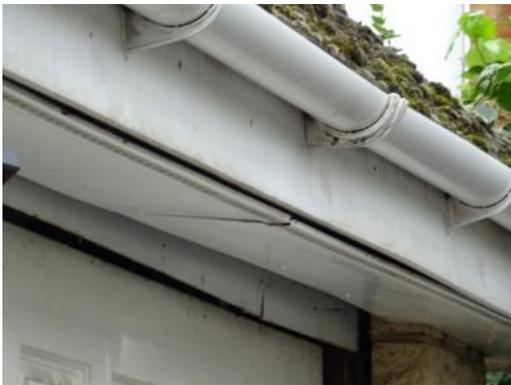
It should be noted that the original soffits may be concealed by the uPVC which may have been formed in fibrous boarding which should not be considered unusual for the age of the property. Therefore prior to any works being carried out to the soffits, we would advise that investigations for asbestos are carried out to prevent any disturbance.
