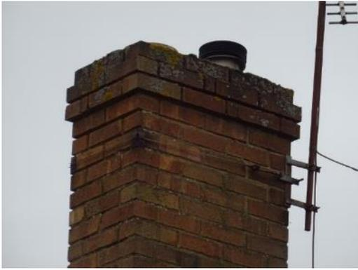
A clay chimney pot is evident to the left hand side of the stack with no significant damage noted. We would advise that the supporting mortar is checked and renewed as necessary when high level access is next provided.
