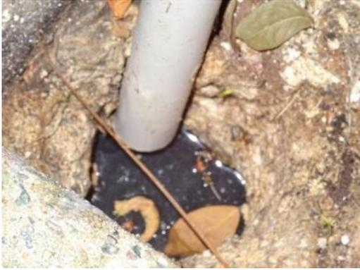
The left hand wastepipe discharged over an open clay gully which was noted to be heavily blocked at the time of our inspection requiring clearing in the immediate term.
