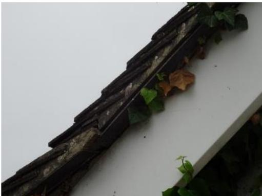
The fascias are uPVC which are noted to be in a serviceable condition having been firmly secured into position however require cleaning down.
