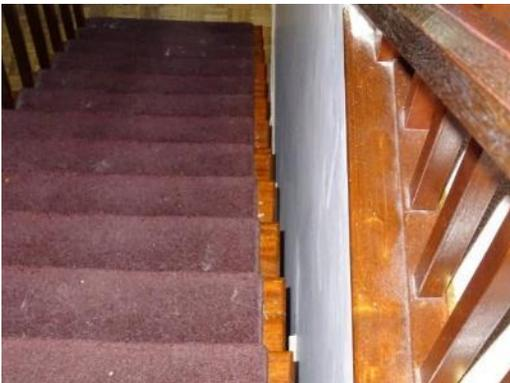
The stairs and landing has been covered with a fully fitted carpet and generally felt level and firm underfoot. Various floorboards were noted to creak underfoot which we would advise are secured down with either serrated nails or screws when the carpet finishes are next pulled back.
