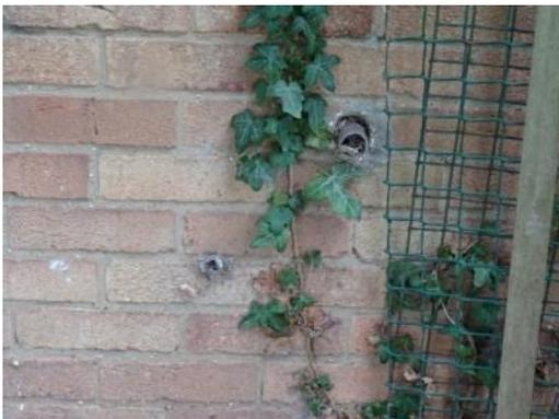
A significant vine was growing up the elevation. Due to the extent of the root system we would advise that this is removed in order to prevent being a risk to the foundations and adjacent drainage.
